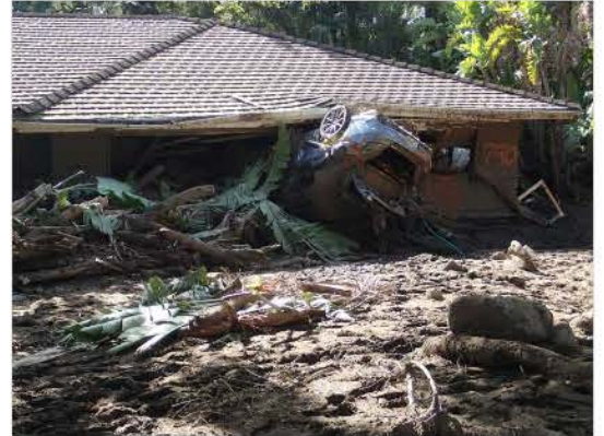
The aftermath of the January 9, 2018 debris flows in Montecito, California.
